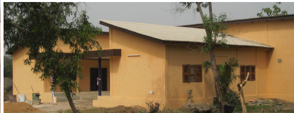
The new dormitory block in Bonou
