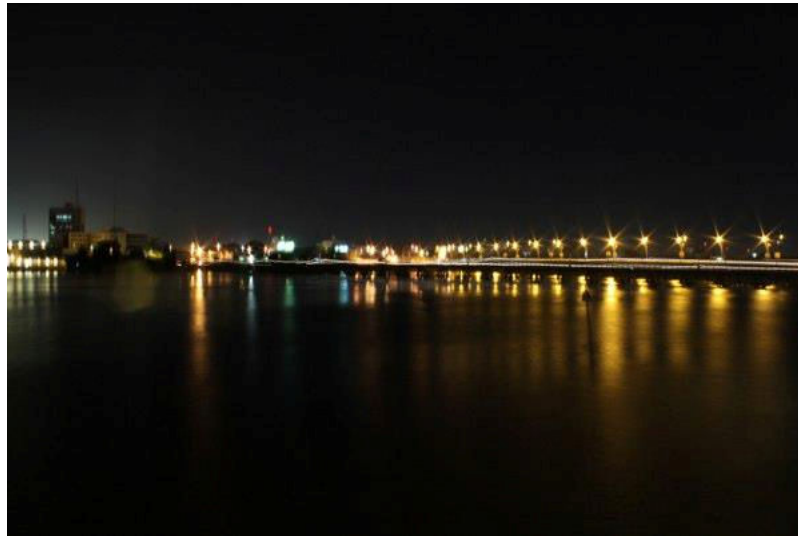
One of the 3 bridges on the Nokoué Lake in Cotonou
